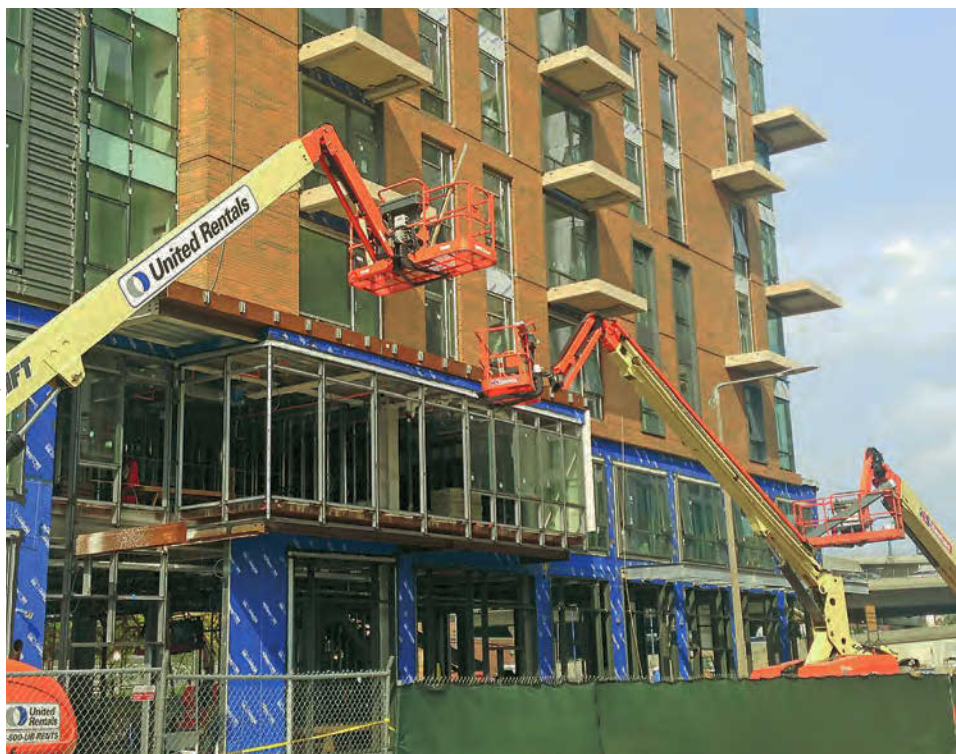
Ink Block construction site at 300 Harrison Avenue.
